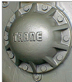
Original oil pressure sensing port.
